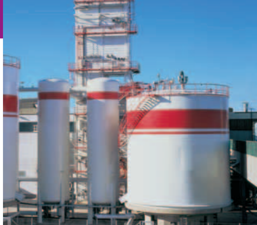
High performance protection for silos and tanks is carried out with an epoxy-polyurethane coating system.
