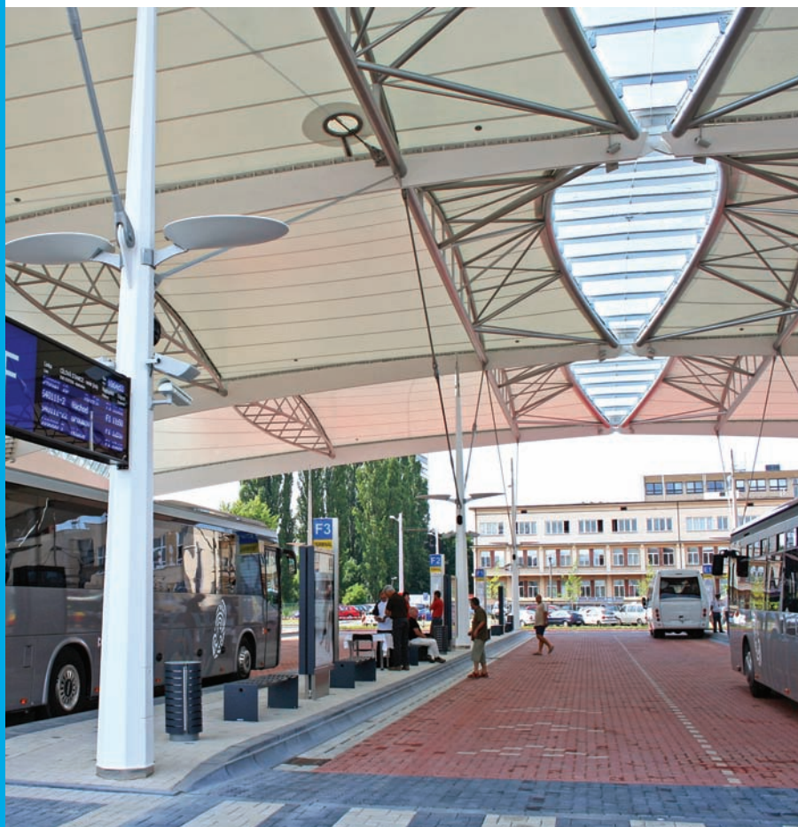
Terminal of public transport, Hradec Kralove, Czech Republic.
