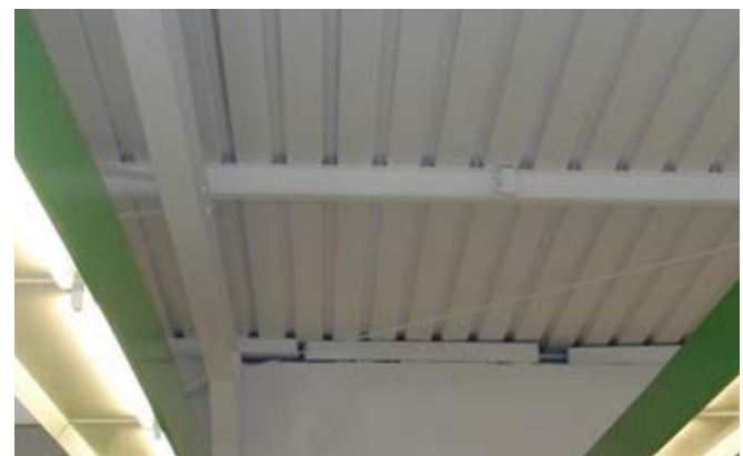
GrafoTherm anti-condensation coating on a roof plate
